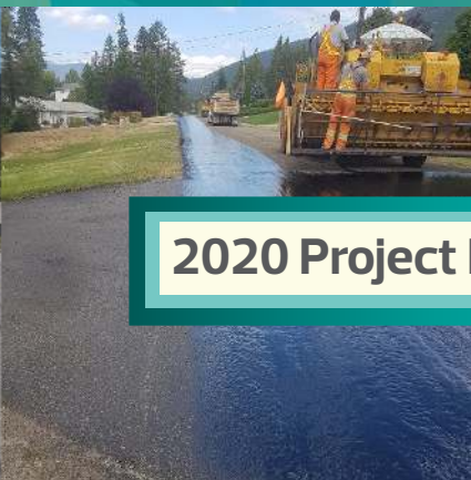
Chip Sealing 1st Ave NW
