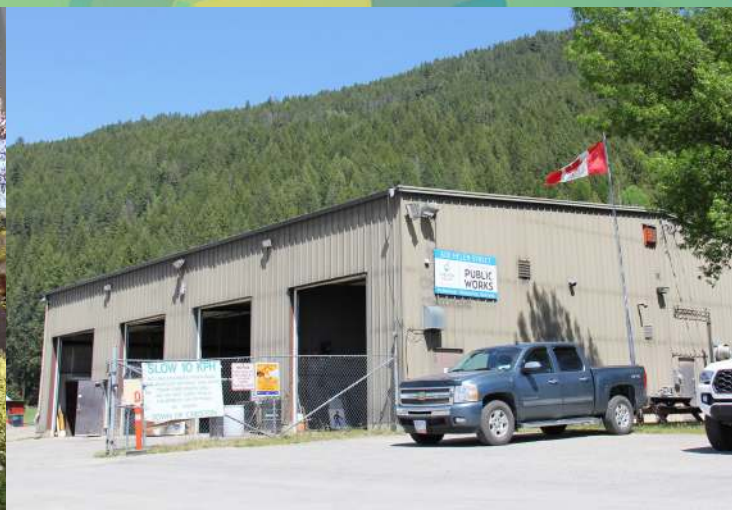
Public Works Building
